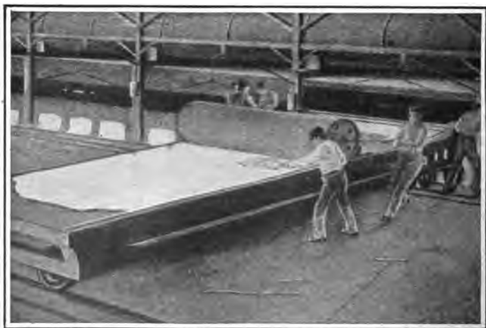
FIG. 90.—Rolling plate glass. (Permission of Scientific American .)
